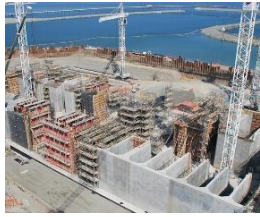
Sohar Seawater Intake Pumping Station
