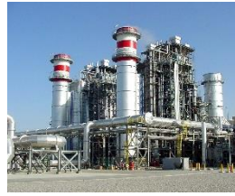
Barka Power & Desalination Plant
