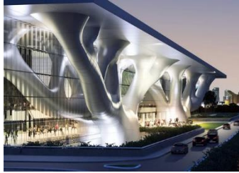
Convention center, Qatar (LEED Gold)
