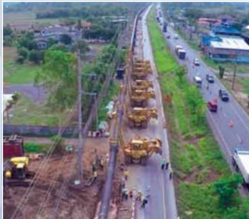
Fourth Transmission Pipeline EPC2 - Thailand
