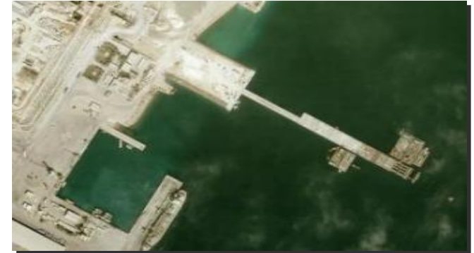
QATALUM PROJECT JETTY AND SEAWATER INTAKE AT MESSAIEED
