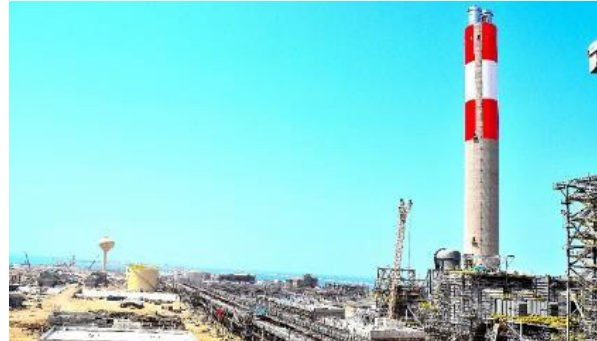
SHUQAIQ STEAM POWER PLANT (2400 MW), JEDDAH
