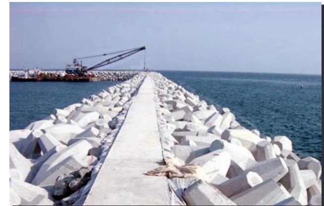
HALUL HARBOUR REFURBISHMENT PHASE I, NORTH QUAY AND WEST BREAKWATER
