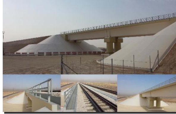
DOUBLING OF DAMMAM-HOFUF MAIN LINE
