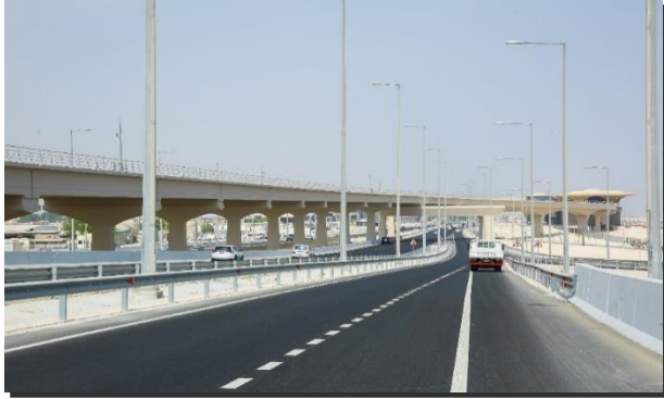
DESIGN & BUILD PACKAGE - RED LINE SOUTH ELEVATED & AT-GRADE, DOHA
