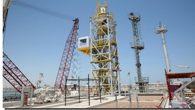
EPIC FOR BERTH & PORT INFRASTRUCTURE FOR RLPEP PHASE 2, RAS LAFFAN
