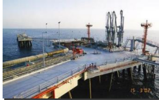
NEW TANKER TERMINAL FOR SHOAIBA DESALINATION PLANT, SHOAIBA
