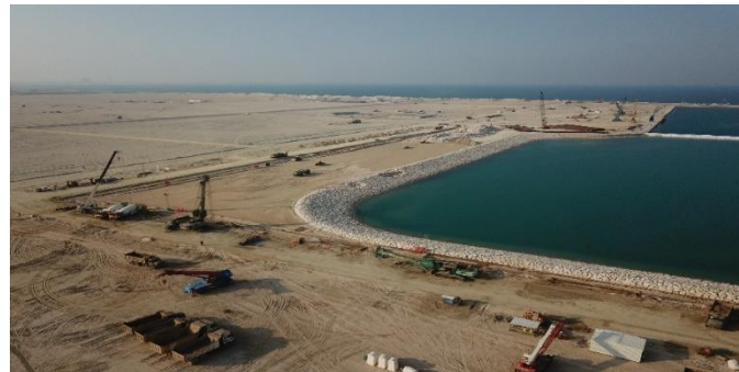
DREDGING, RECLAMATION AND MARINE STRUCTURES PACKAGE AT KING SALMAN , RAS AL-KHAIR
