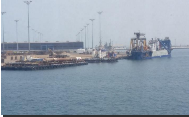
IMPROVEMENT AND EXPANSION OF MARINE FACILITIES AT PORT OF FARASAN
