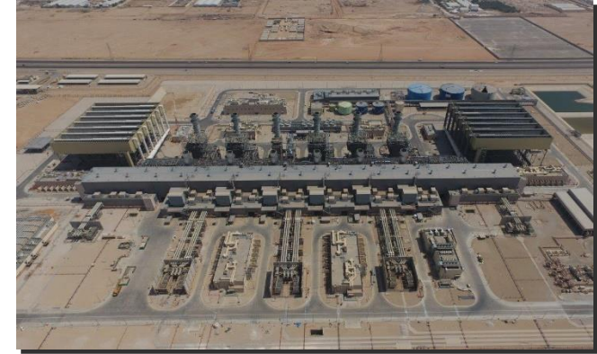
EARLY AND CIVIL WORKS AT POWER PLANT PP14 (1,650 – 1,950 MW), RIYADH
