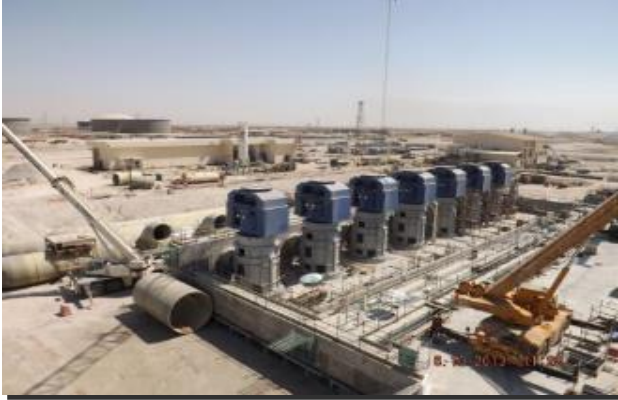
YANBU 2 POWER AND WATER PROJECT (600 MW), MARINE FACILITIES, YANBU
