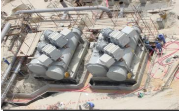
EPC CONTRACT FOR METHANOL PLANT REVAMP AT MESAIEED
