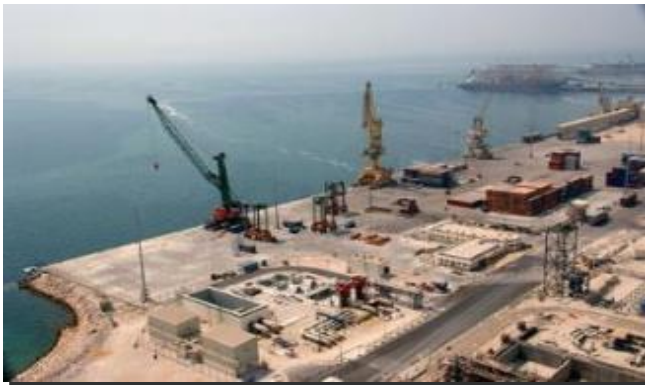
ENGINEERING, PROCUREMENT, SUPPLY, CONSTRUCTION & COMMISSIONING OF THE MESSAIEED POLYETHELENE QATOFIN PROJECT-MARINE WORKS
