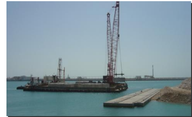
PEARL GTL PROJECT, CONSTRUCTION OF MATERIAL OFFLOADING FACILITY, RAS LAFFAN
