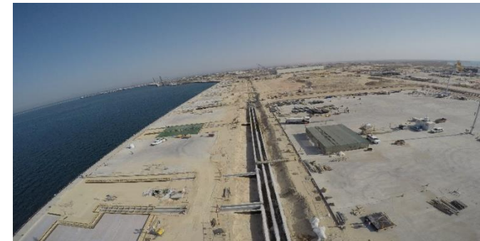
UPGRADE PIER FACILITIES AT TANAJIB
