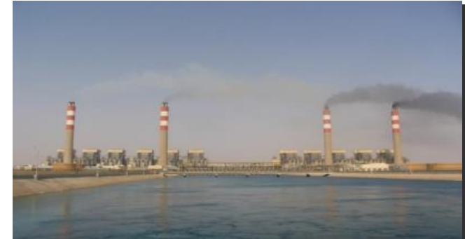
SHOAIBA POWER PLANT STAGES I, II, III (6.1 GW)
