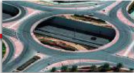
Ras Abu Abboud Tunnel
