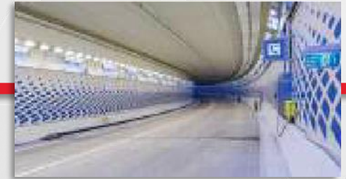
Lusail Expressway Tunnels
