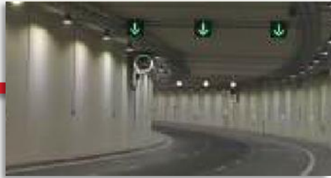
Mall of Qatar Tunnel
