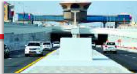
Al Wakrah Tunnel
