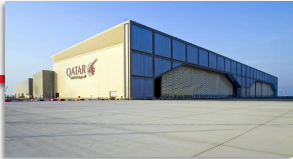
Air Maintenance Hangar Complex
